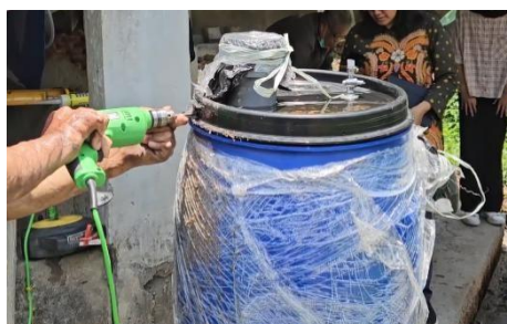
Gambar 3. Proses Perakitan Biogas Digester
